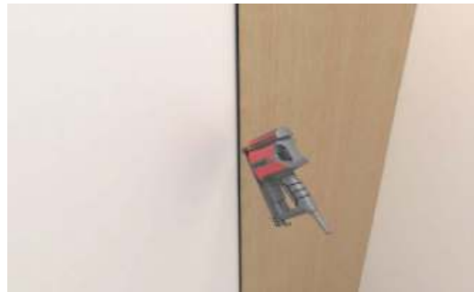
4. Insert the metal trim into the groove from the side of the panel, and then nail the trim to the wall.
