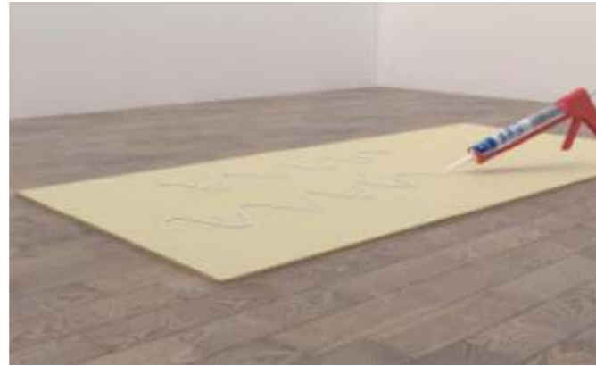
2. Put nail - free glue on the back of the wall panel.
